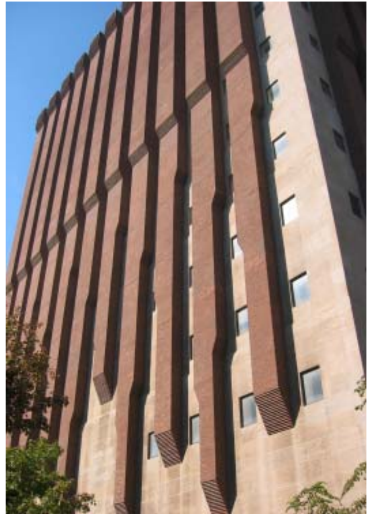
Figure 1-The distinctive concrete columns on the exterior of the building, which house the original lab exhaust riser, presented many challenges to the renovation of the exhaust system.
